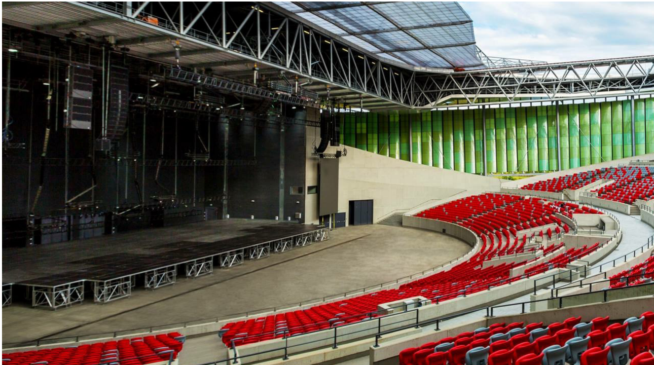
Photo: Scenos Techninis Servisas, Black Sea Arena, Georgia.
